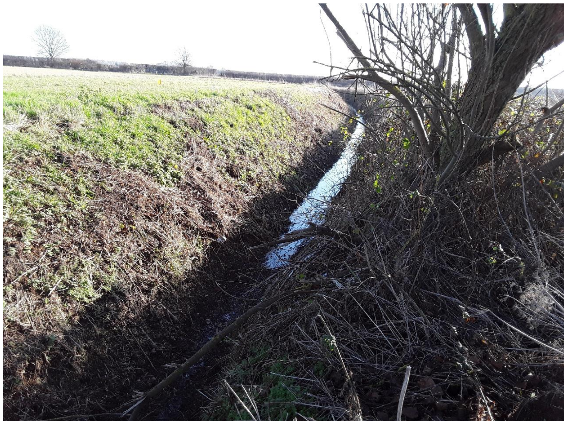
Photo 10 – 5m deep by 5m wide drain with 0.2m of lying water
