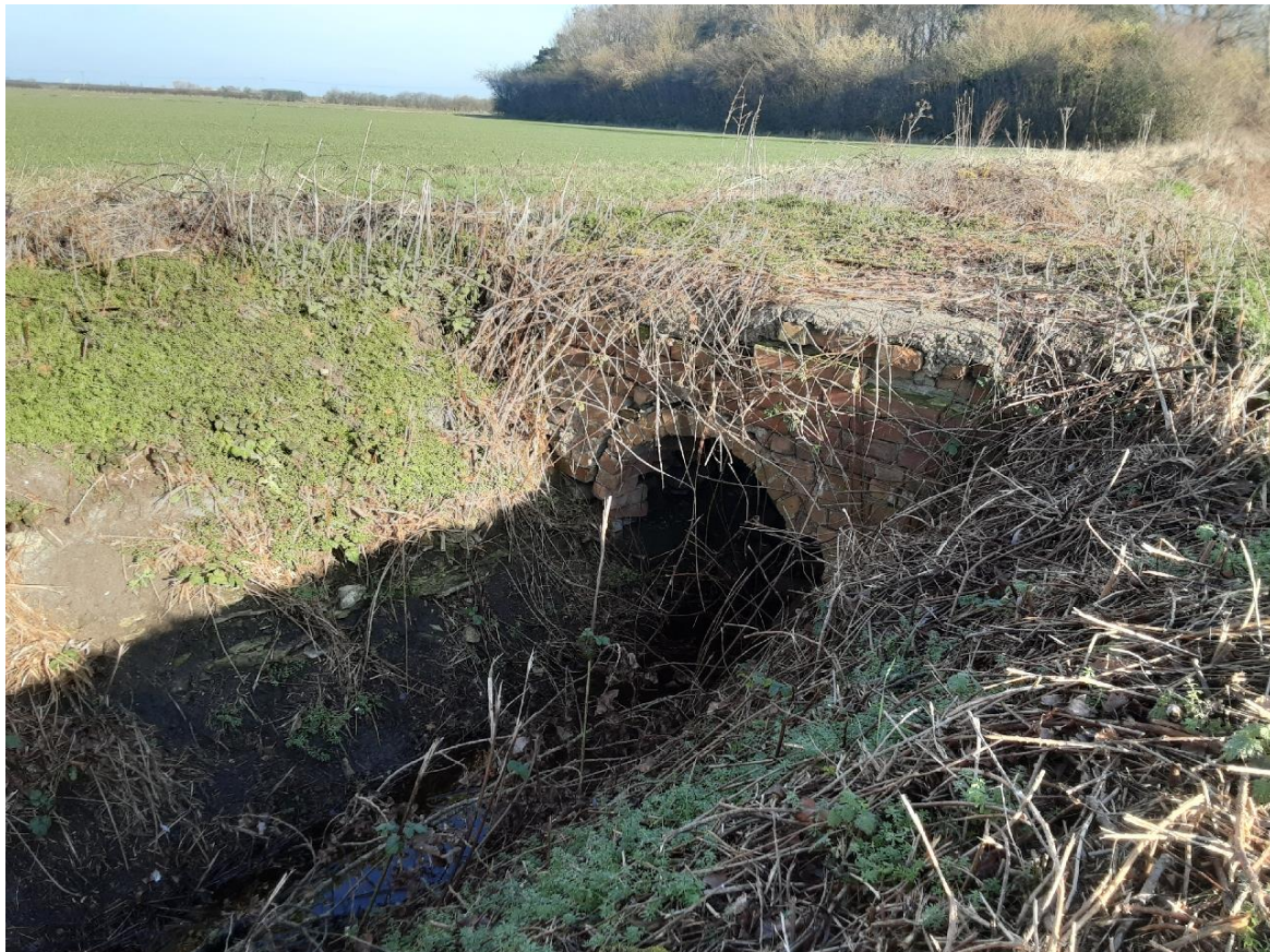
Photo 18 – 1.5m diameter culvert
