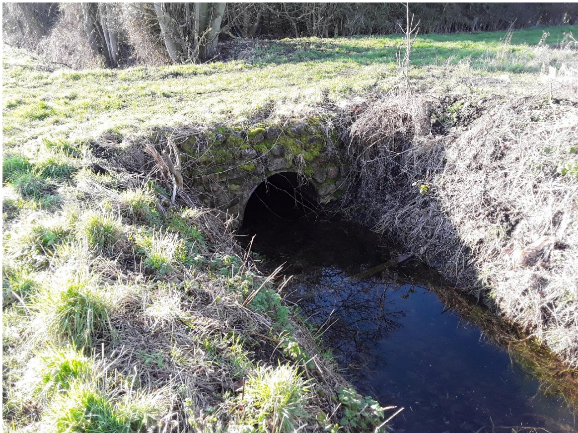
Photo 16 – 1.5m diameter culvert
