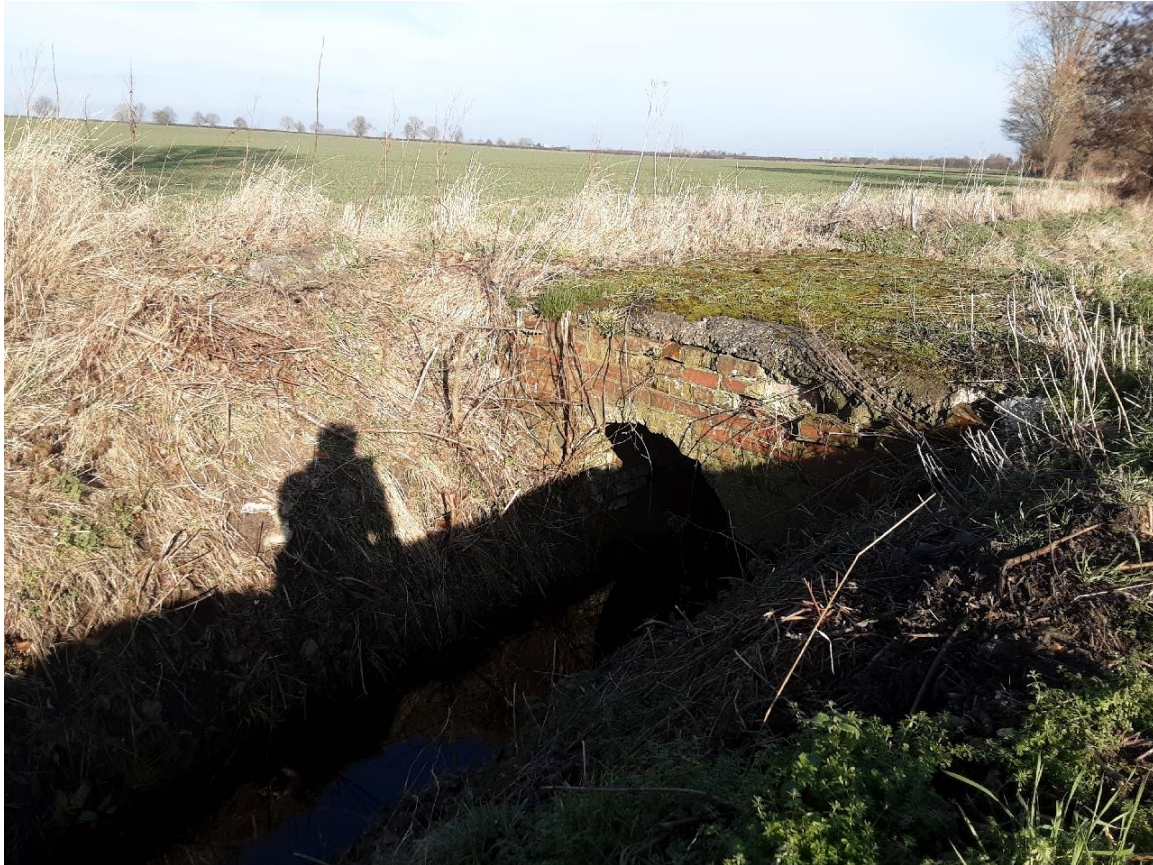
Photo 19 – 1.5m diameter culvert
