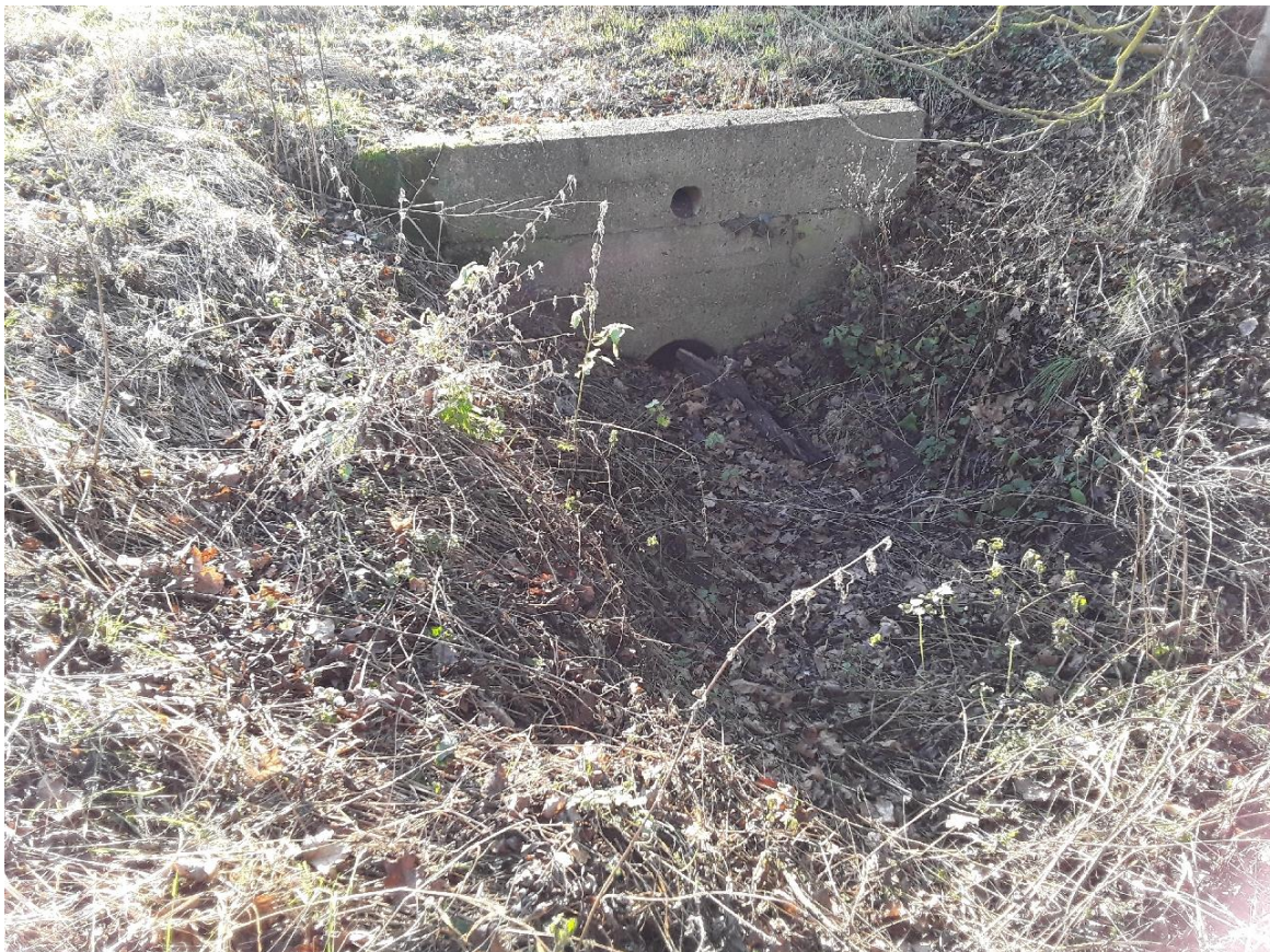
Photo 4 – 0.5m diameter culvert
